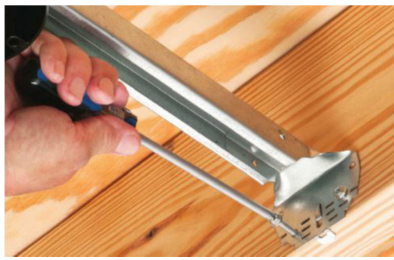
Bracket mounts securely to joists.
