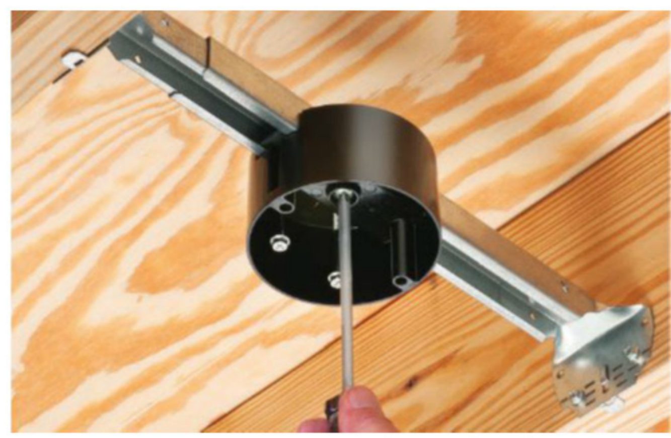
Loosen center screw to position box on bracket.
