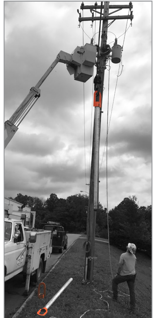
Conduit stays level for connection.
