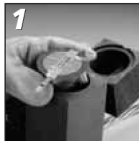
1 Insert CADWELD PLUS package into mould
