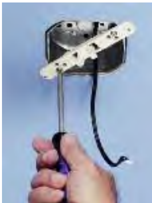
Attach SC5 bracket to inside of the box.
